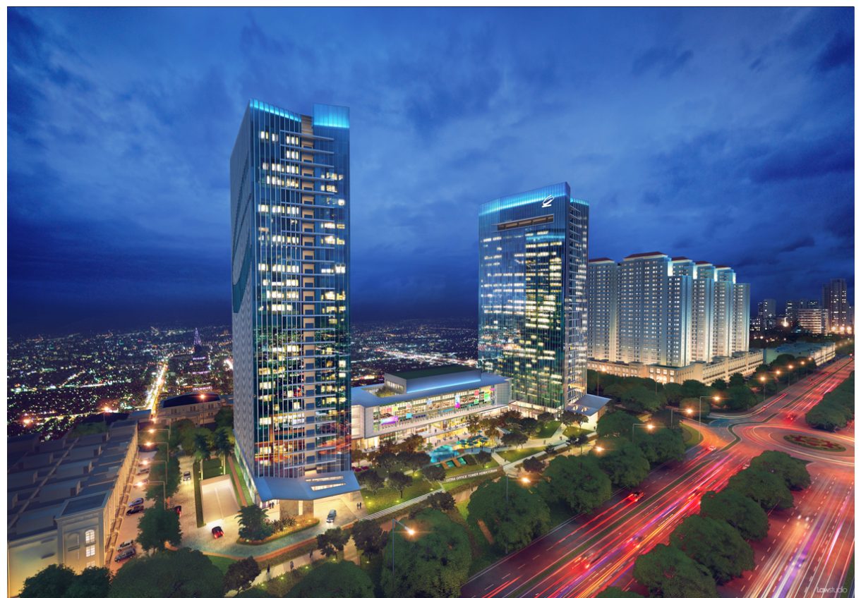
The Citra Towers Kemayoran are located in Jakarta and have received a preliminary EDGE certificate from the Green Building Council Indonesia. The mixed-use complex features a pair of 24-story office towers, a 23-story apartment building and a five-story retail podium.
